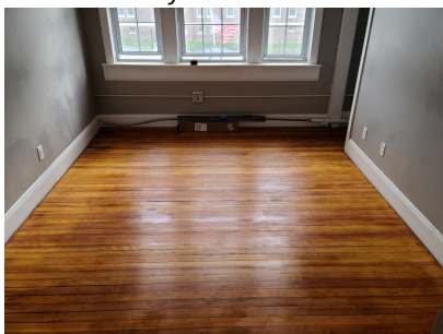
3 - Floor refinished, drywall and trim installed and painted
